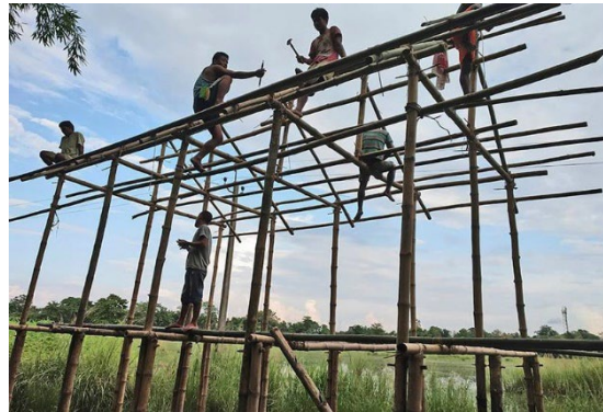
Figure 23. Assembling Cross Bracing (SEEDs)
