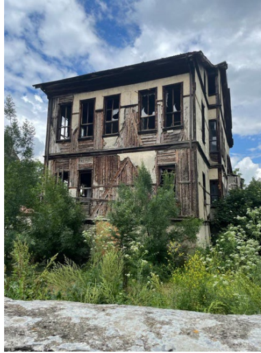
Figure 7. Wooden Construction of a Mudurnu House
