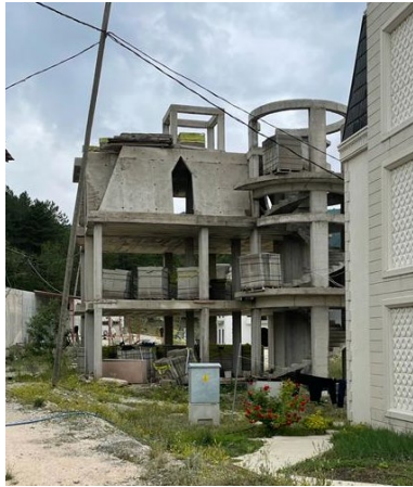
Figure 8. The reinforced concrete structure of a typical villa in the Burj al Babas project
